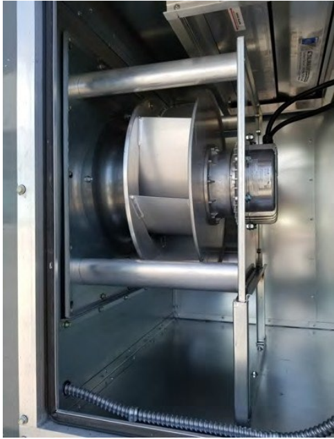
Electronically Commutated Motor (ECM)
